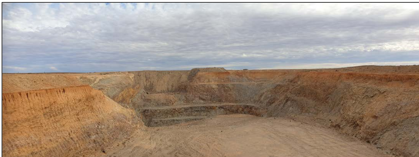
Figure 8: Existing shallow Vertigo Pit facing south west, mineralisation extends gently downward from the south eastern (left) side of the pit.
