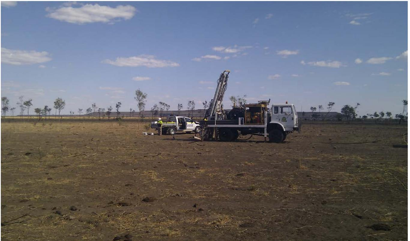
**Figure 2:** First hole of aircore grid drilling program at FC4S Sevastopol graphite project. Ernest Henry mine waste dumps visible in the background.
